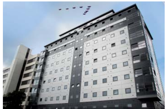
Pictured: External view of Lyme Regis House with the Red Arrows flying over
